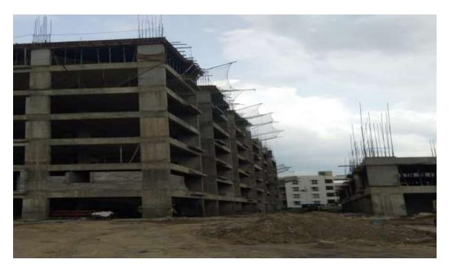
Block B2: Second Floor slab 1<sup>st</sup> Half concrete completed & in 2<sup>nd</sup> half portion slab shuttering & barbending works are on progress.
