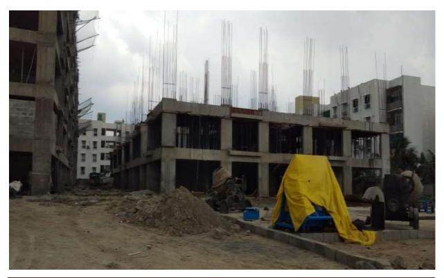
Block C1: Sixth Floor slab completed & in Seventh Floor slab Suttering & Barbending works are on progress
