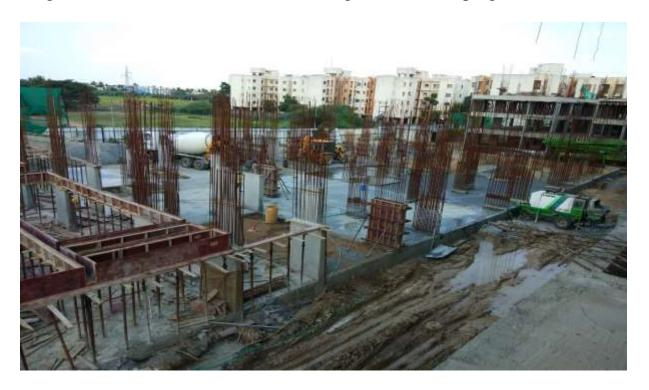
Block D2 : Sixth Floor slab  $1^{\rm st}$  Half Portion Shuttering & Barbending works are on progress.
