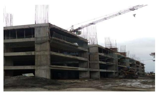
Block C3: Second Floor 1<sup>st</sup> Half concrete completed & in 2<sup>nd</sup> half portion shuttering works are on progress. In Third Floor 1<sup>st</sup> Half Slab Shuttering & Barbending works on progress
