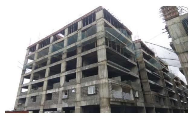
Block C2: Fourth Floor slab 1<sup>st</sup> Half concrete completed & in 2<sup>nd</sup> half portion slab shuttering & barbending works are on progress.
