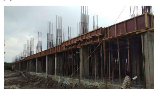
Block A2: First Floor Slab shuttering & barbending works are on progress.
