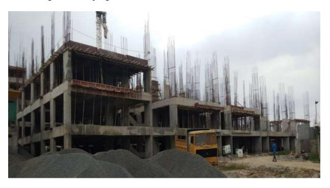
Block D1: Pile Cap Works Complete. Earthwork backfilling & PCC for on Progress. First Floor 1st Half Slab Shuttering works are on progress.
