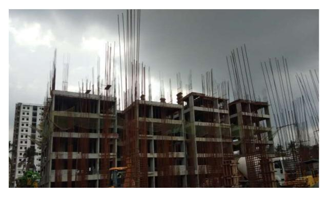
Block D3: Fourth Floor slab 1<sup>st</sup> Half Portion Shuttering & Barbending works are on progress.
