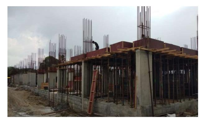
Block B1: Sixth Floor slab completed & in Seventh Floor slab Suttering & Barbending works are on progress
